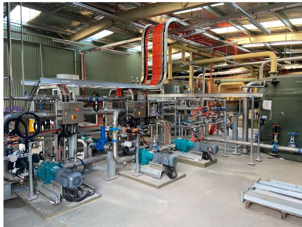
The new Tanker Receiving Facility accepts waste from external septic trucks. The product is then treated and recycled on site.
