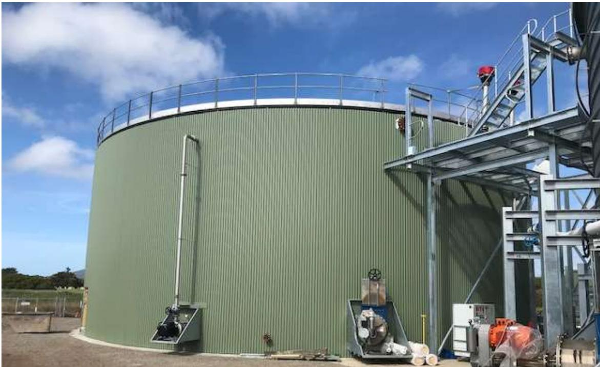
Anerobic digester with cladding
