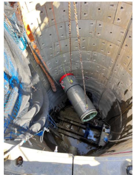
Tunnel boring machine being prepared to launch towards Worksite 1.
