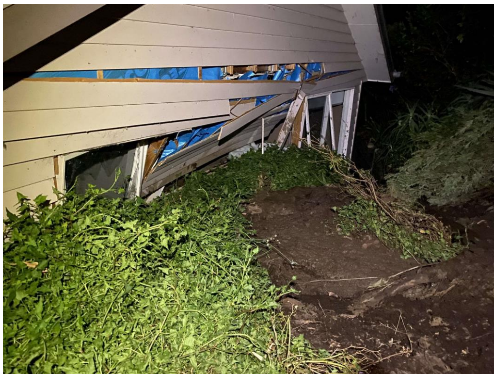
Figure 52: Photograph taken on the night of 5-6 January 2025 showing landslide debris against rear wall of 3 Penny Lane
