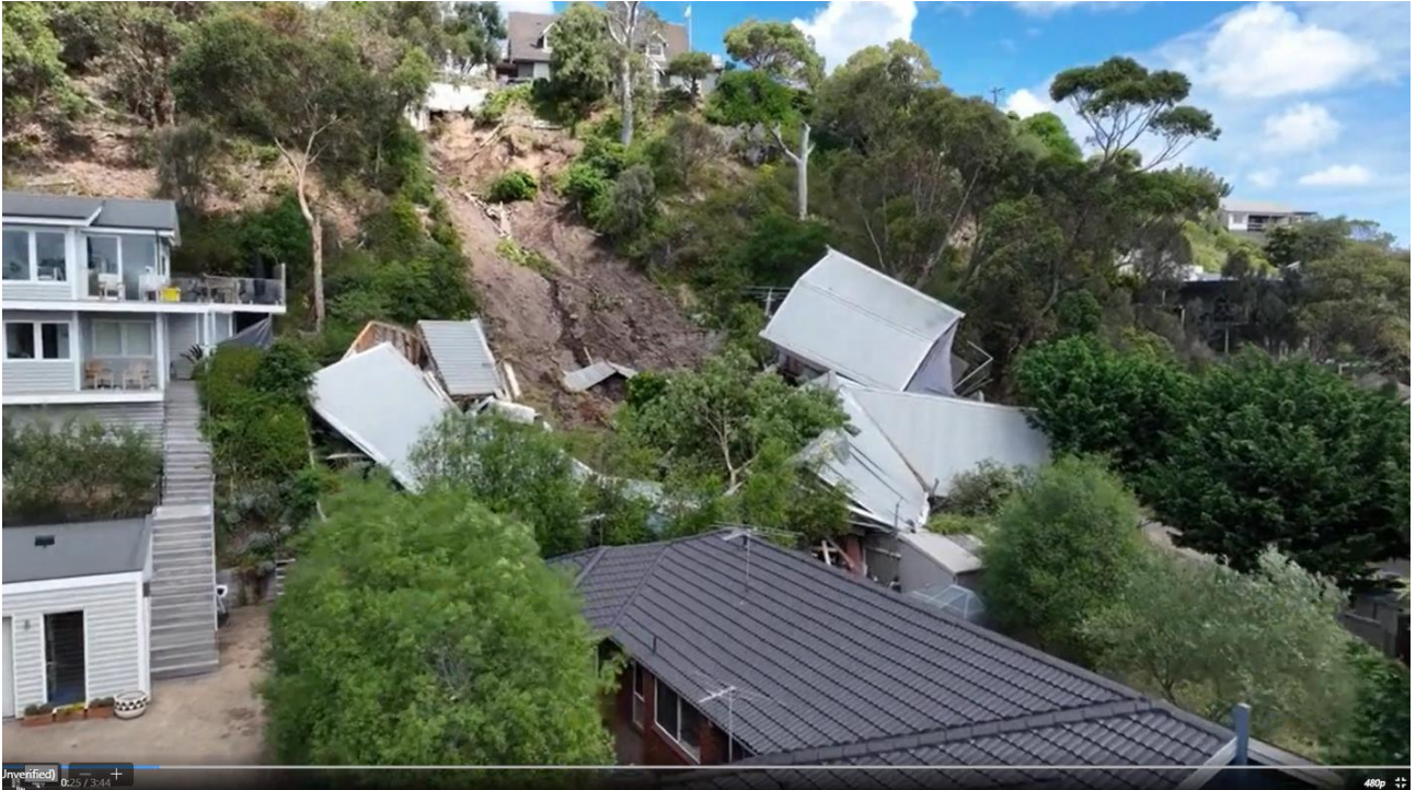
Figure 10: Drone footage taken from toe of slope failure showing the gully, denuded by slipping debris from upslope.
