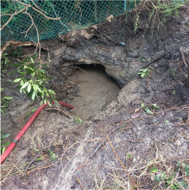
Figure 45: Provided by SEW, understood to have been taken on 31 December 2024, showing the ground collapsing during water pumping at Bayview Road leak site. Hole assumed to have been excavated by small excavator on site at the time.
